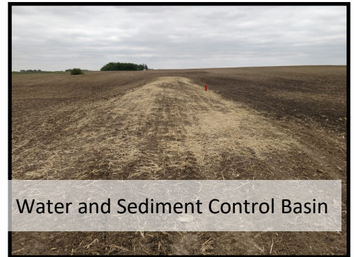
175' earthen embankment with a 48" concrete structure
