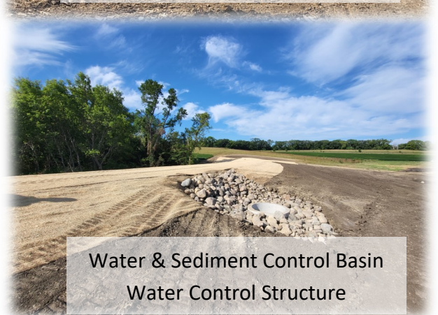
Water and Sediment Basin/Terrace Repair
