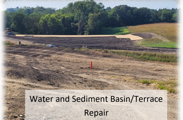
Water & Sediment Control Basin
