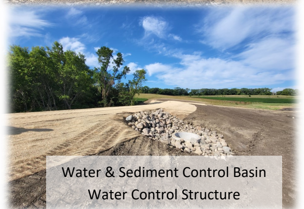
Water and Sediment Basin/Terrace Repair
