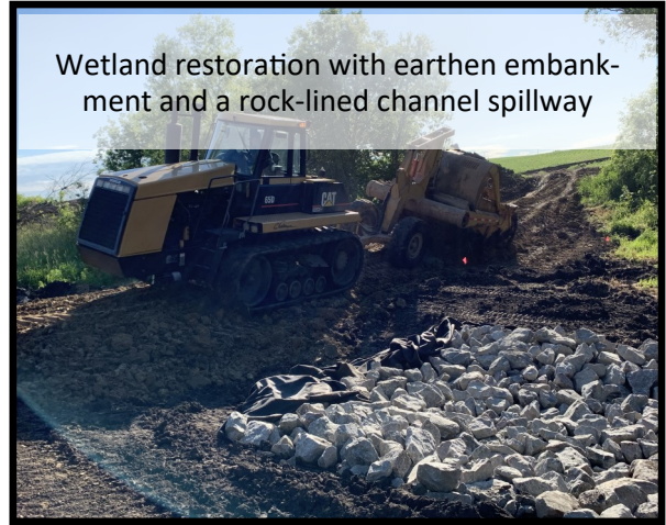
Wetland restoration with earthen embankment and a rock-lined channel spillway
