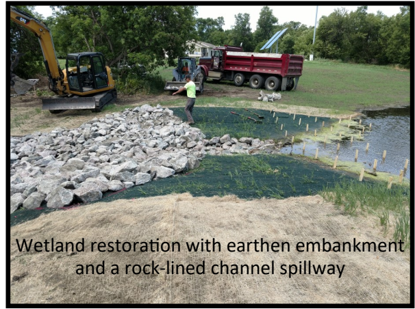
Wetland restoration with earthen embankment and a rock-lined channel spillway
